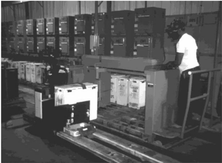
Figure 29. A battery-charging station, designed to reduce floor space for this operation, freeing up more area for slots.
